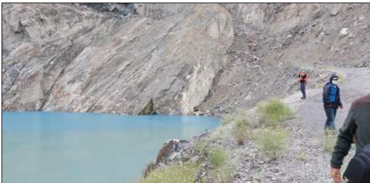
Figure 7.11: Intake Area view from Upstream of Weir, Sound Rock Exposed
