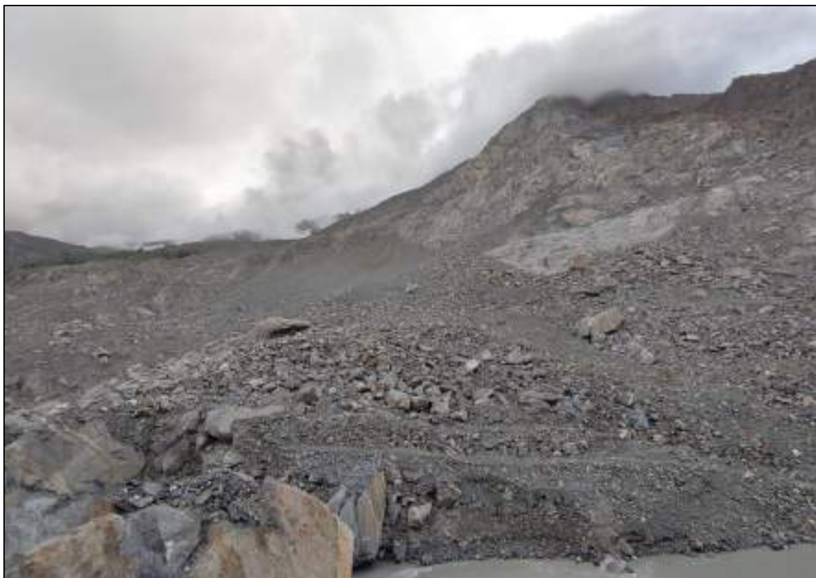
Figure 7.8: Right Abutment view from Left Abutment, Slide Mound of ABGM
