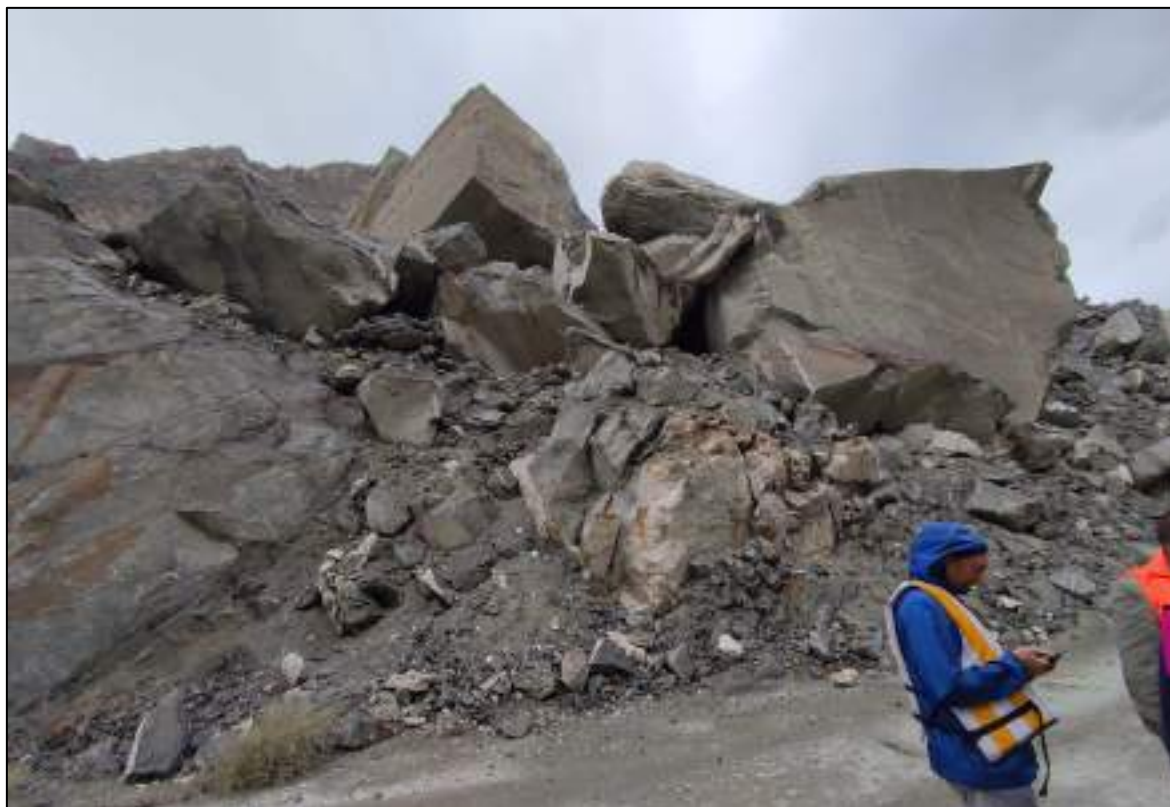
Figure 7.9: Left Abutment view on side track, Large size Boulders from slide material
