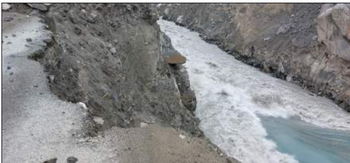
Figure 7.10: Left Abutment, Fresh Slide area and completely damaged walkway / path towards chute area
