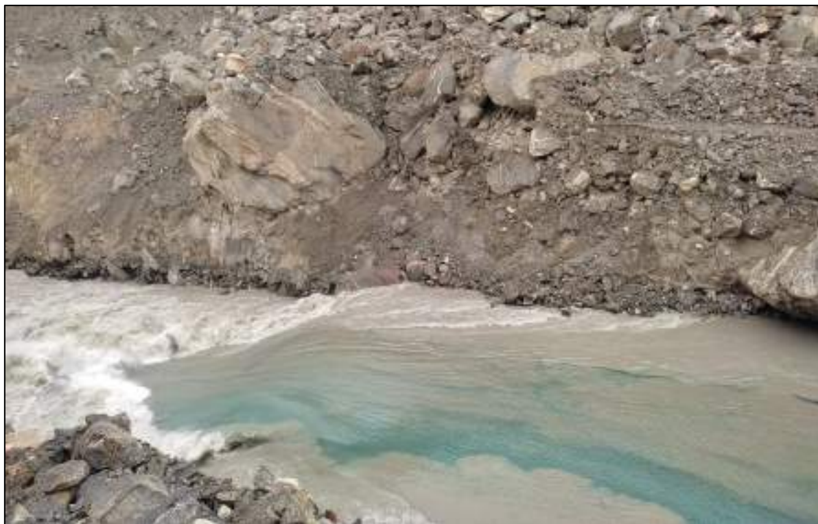
Figure 7.7: Excavated Spillway view from Weir Axis
