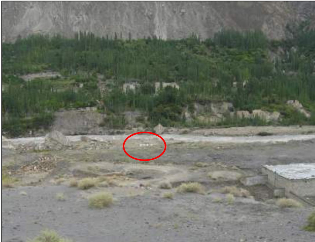
Figure 7.13: Marked Power House Area near Left Bank Hunza River, Overburden visible along the Penstock Alignment
