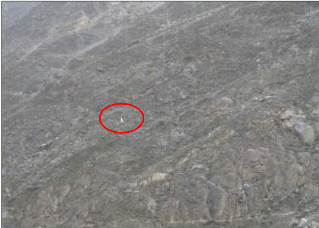
Figure 7.12: Flagged Surge shaft Area, Sheared and Jointed Rock Exposed
